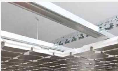
Installation of metal structure with 300 mm pitch
