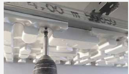
Installation and fitting of head panels on the metal support structure with 35 mm screws
