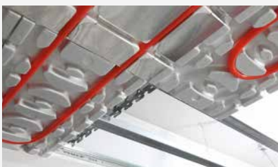
Installation and fitting of R883-1 panels and pipes along the preformed panel and head housings
